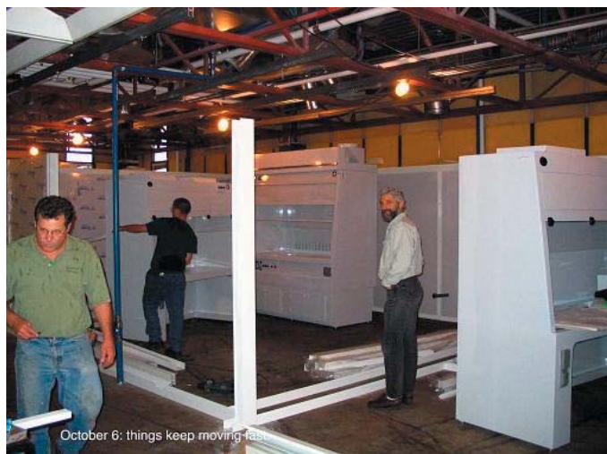
Constructing the new labs in EOS
